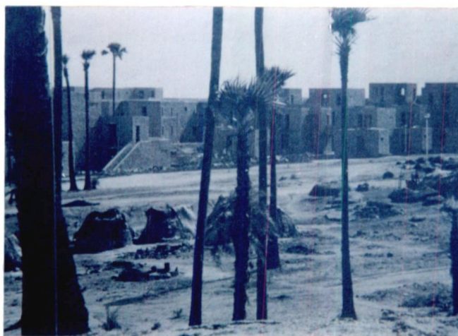
Fig 15 ; mixed income housing, Hyderabad, India by Balkrishna Doshi - 1976
