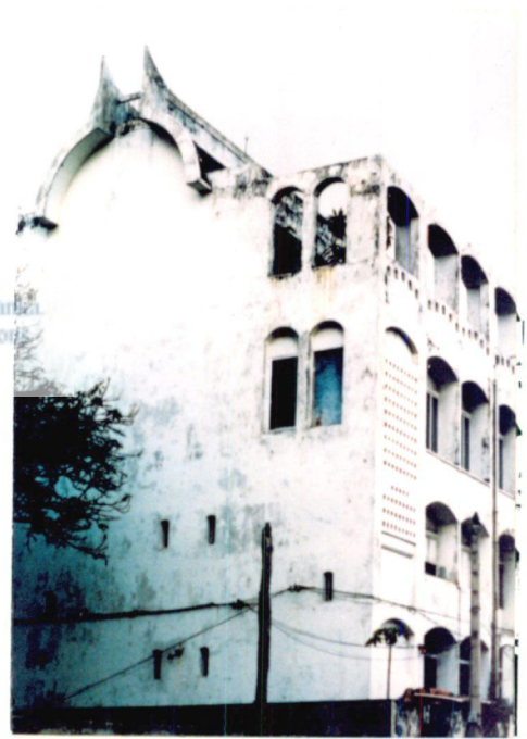
Fig 58 ; Apartment building, Galle Face
