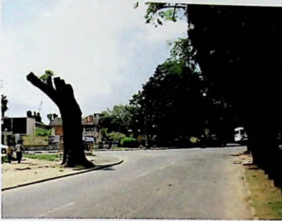
Fig. 3.14 In case of parasitic attacks roadside trees are decay and die. At Baudhaloka mawatha and Wijerama road junction. In old age trees are increasing liable to suffer dieback and decay. Credit: Gunasinghe W. K.D.
