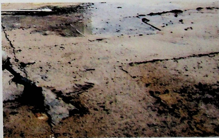
Figure 3.6: Weak adhesion
