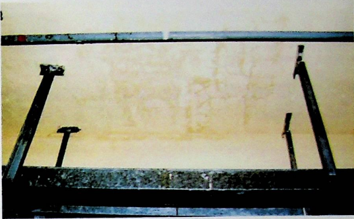
Figure 3.4: Water seepage
