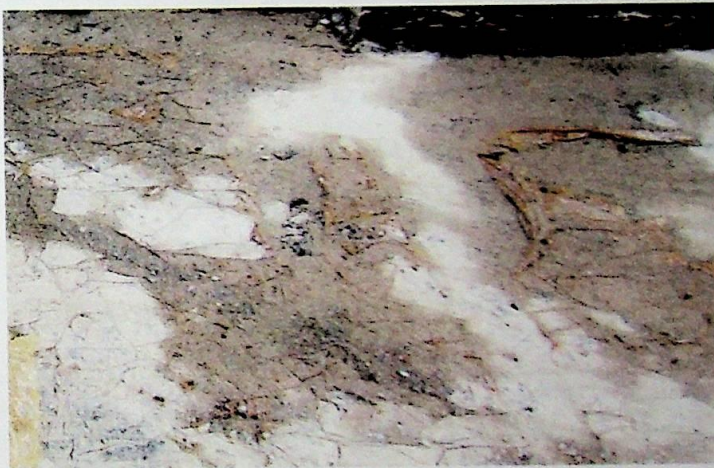
Figure 3.8: Cracked membrane
