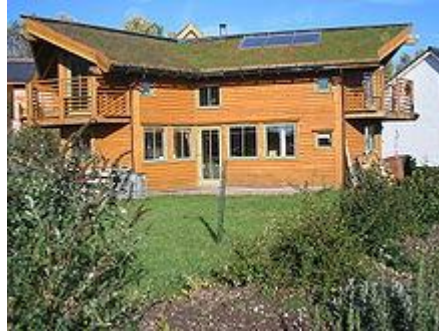
Figure 1 1 An eco-house with a turf roof and solar panels
