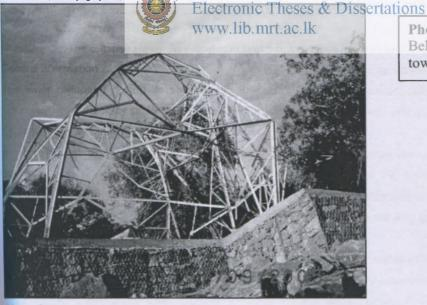
Photo 5.1, Beliatta 70m antenna tower collapse
