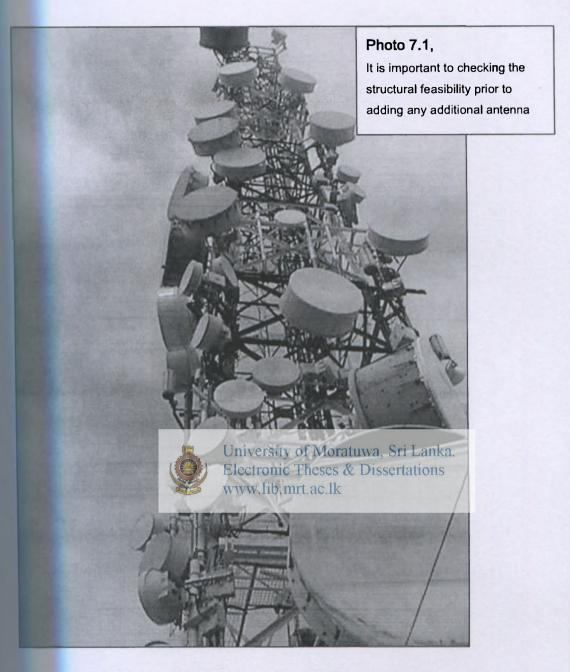
Therefore, it is essential to use accurate method of structural evaluation prior to any change of antenna loads or configuration in steel lattice type antenna structures.
