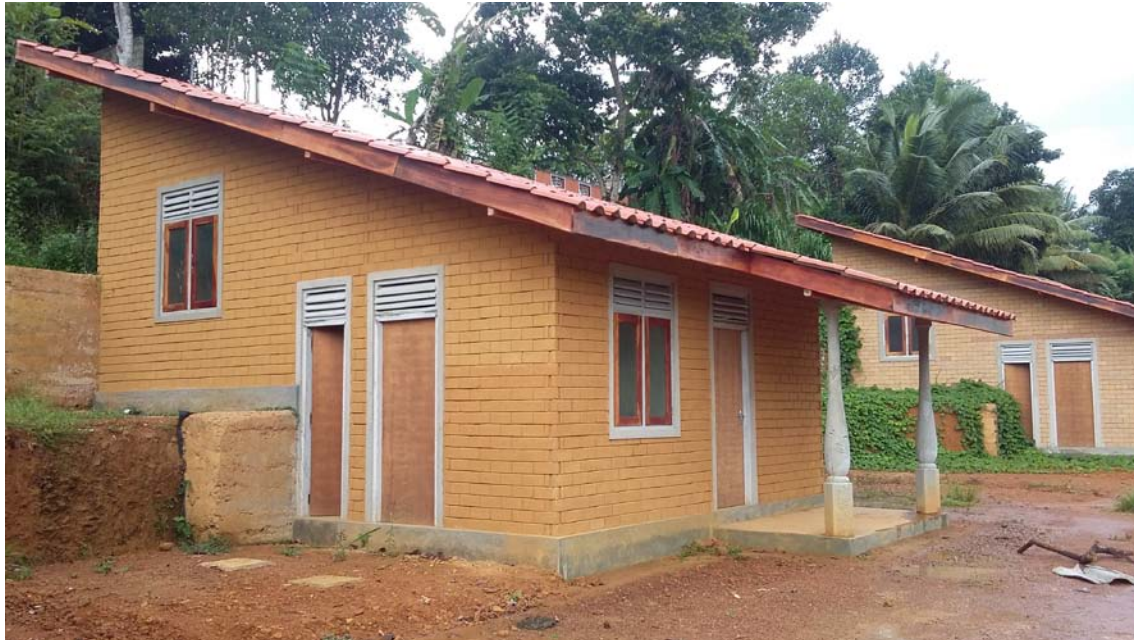
Figure 9: The tiered houses with cement stabilized rammed earth foundations, retaining wall and cement stabilized earth blocks
