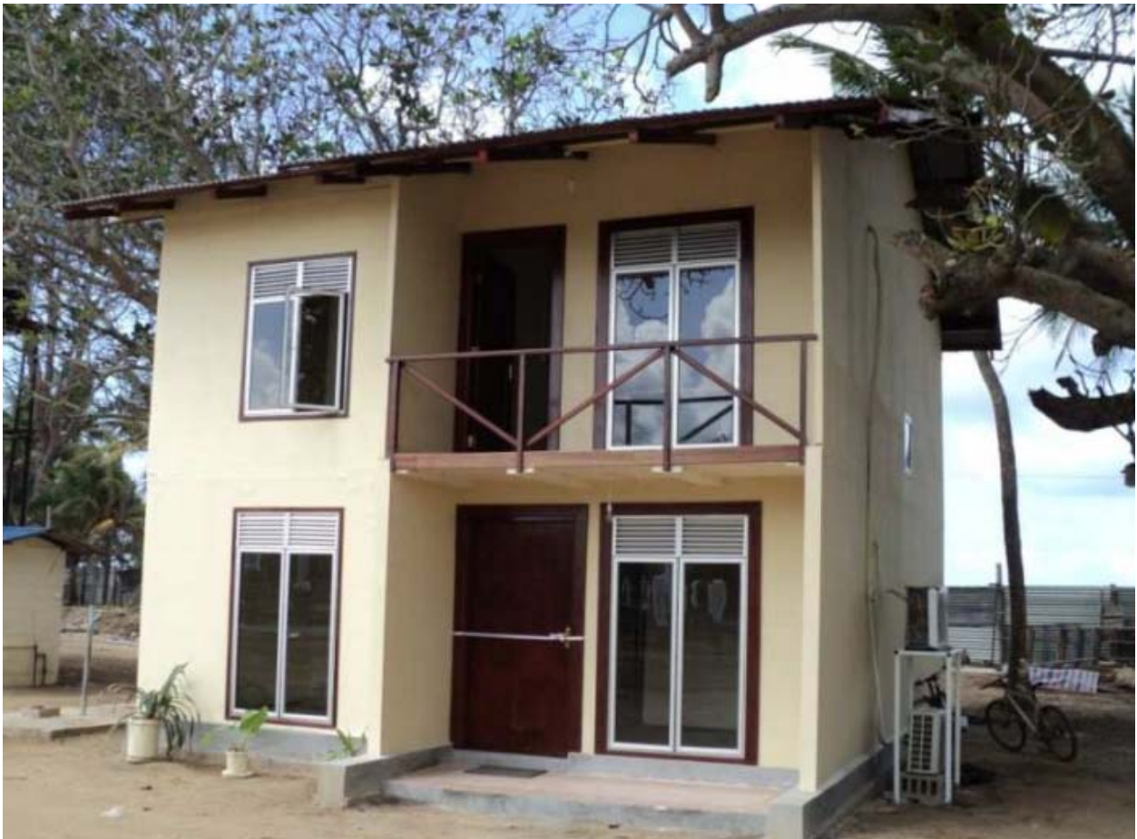
Figure 8: The two storey house with the walls, floors and the ceiling are all out of Durra.
