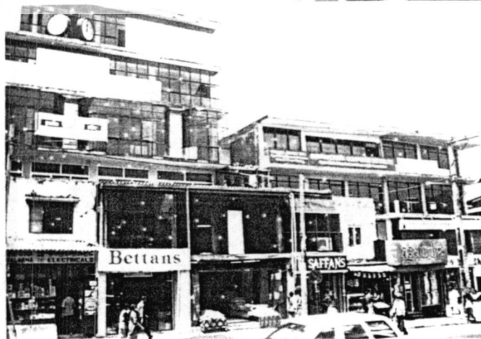
Dense packing of shops with narrow frontages. (Fig. 3.11)
