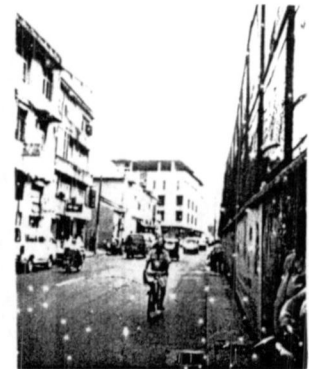
The three to four storey regular skyline and building line makes a group. Start of different character [Fig: 58]
