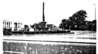
Town Hall; the spatiality of object demanded, to create a unified space [Fig: 68]
