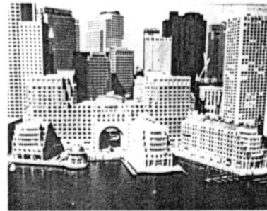
Clear transition from low to high rise buildings [Fig: 43]
