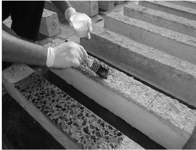
Figure 3.14: Application of primer on beam soffits
