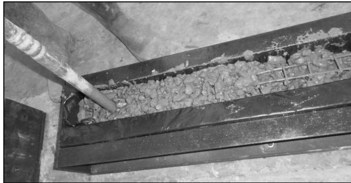
Figure 3.11: Compaction with poker vibrator
