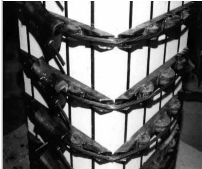
Figure 1.4: Strengthening of a rectangular column with pre-stressed steel (Yarandi et al 2004)
