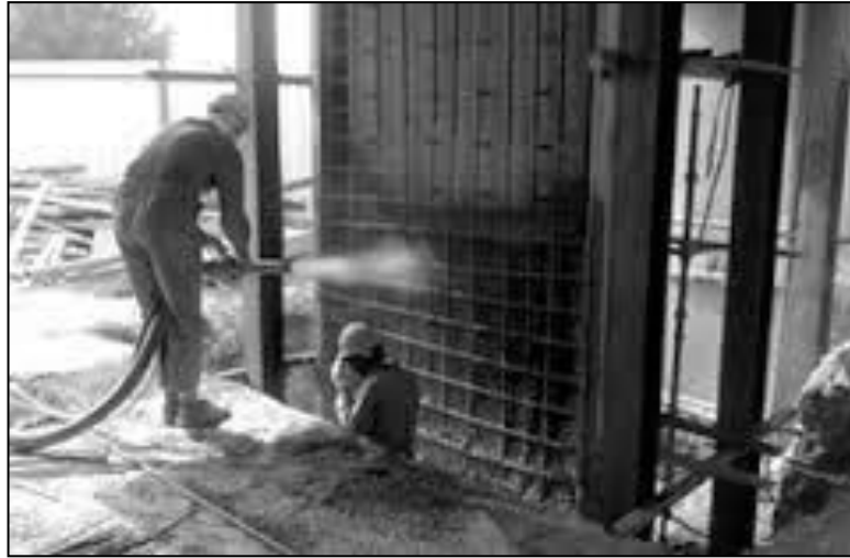
Figure 1.1: Concrete jacketing (Hamara Kuwait commercial division, Viewed December 21 2014 )
