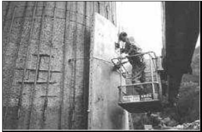
Figure 1.3: Precast concrete jacketing (Dash 2009)
