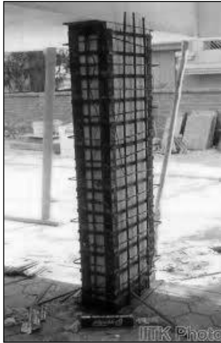
Figure 1.2: Steel jacketing (Reinforced concrete buildings, Viewed December 28 2014.)
