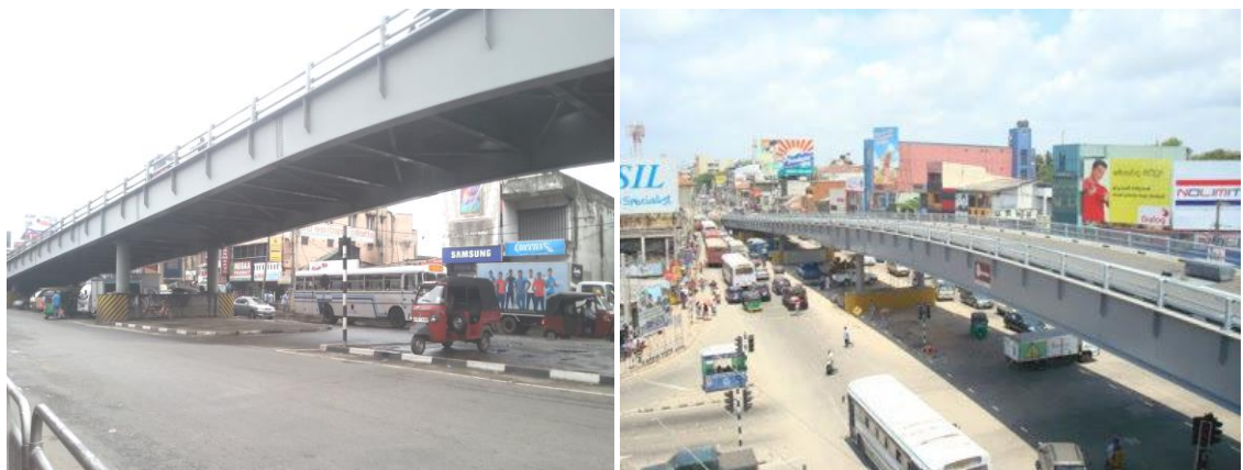
Figure 3.0-24 Dehiwala flyovers and it's underneath space
