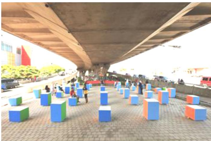
Figure C-6 Parks Pasupati, is a Park located under Pasupati Bridge,
