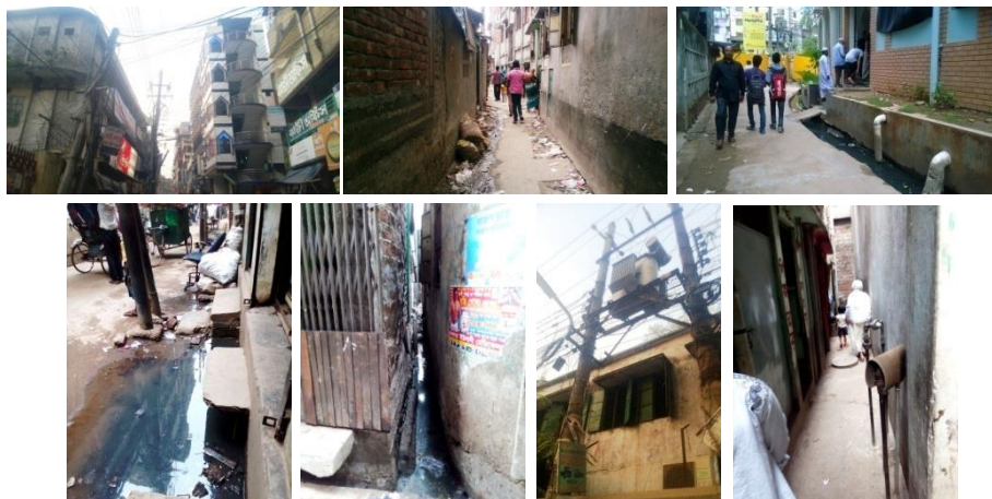
Figure 03: (from left) electric post and wire; narrow road; drainage condition; transformer adjoining buildings; unprotected gas pipes
