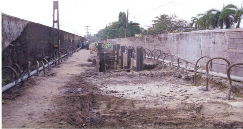
9 PSS- Gravity Pipe Laying [GRP800] at Egodahena Road.
