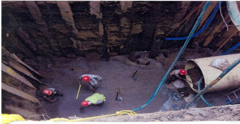
8 WWTP- Gravity Laying T3-T6 [GRP1500] at Treatment Plant Road.
