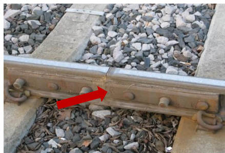
Figure 2.2: 'T' Insulator
