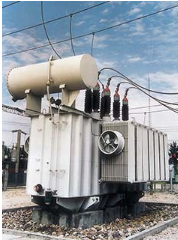
Figure 5.7- Scott -T Transformer
