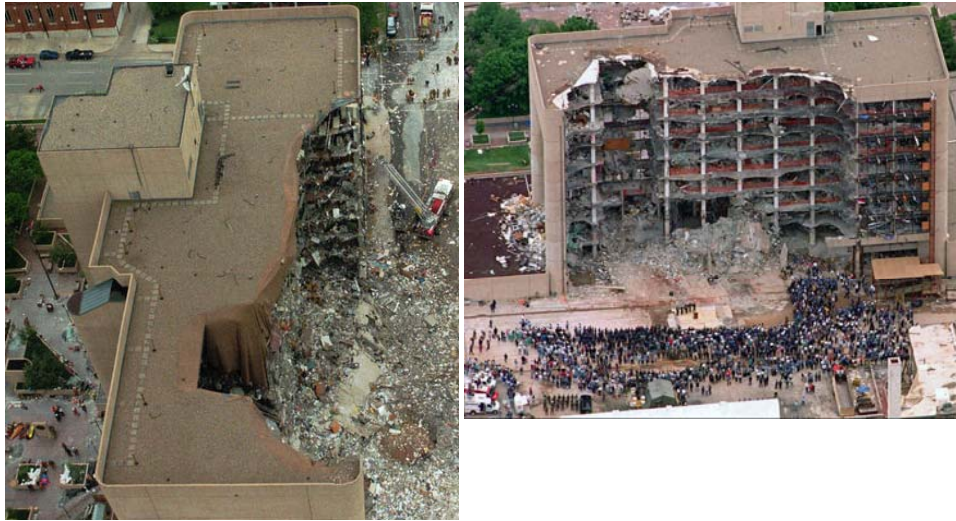
Fig- 1.2 Damages to Murrah Federal Building, Oklahoma City
