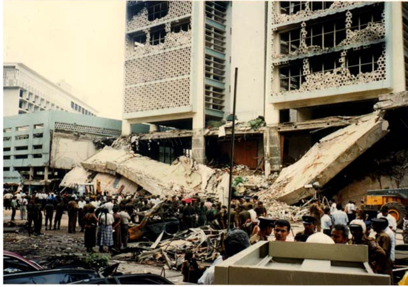
Fig- 1.1 Central Bank Building after the bomb blast
