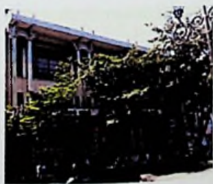
Fig.108 People Bank building Source. Author
