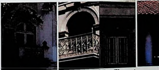
Fig.77 Historic use of colour in Building Elements Source. Author
