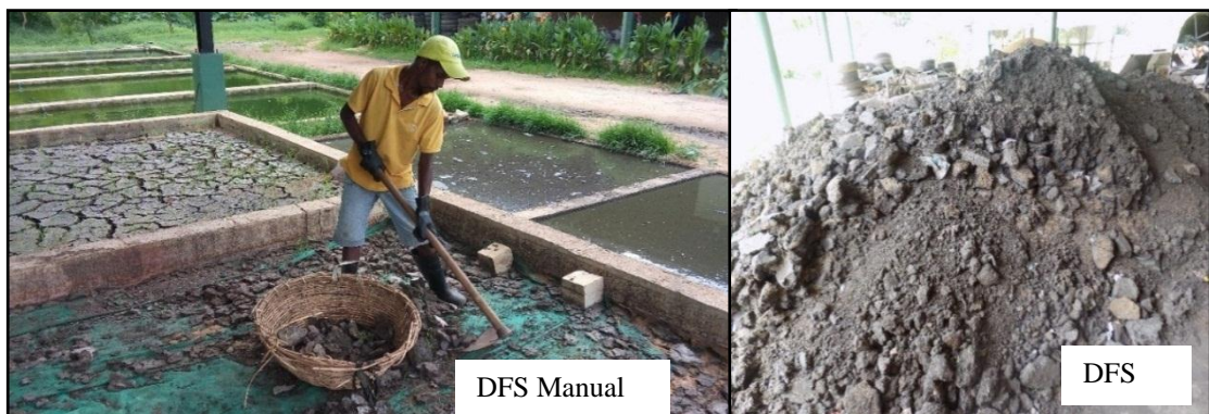
Figure 16 - Manual collection of DFS & DFS pile
