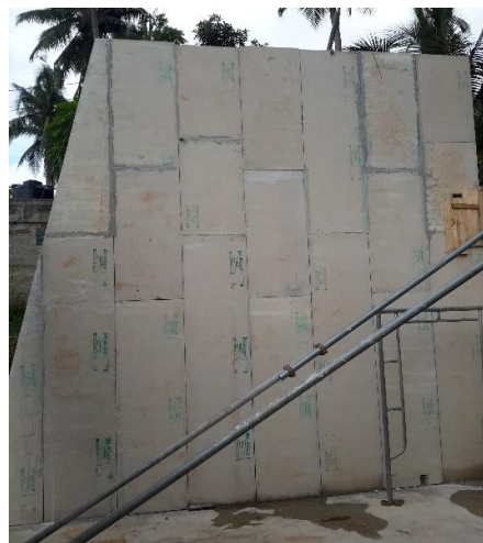
Figure 4-6: Similar house constructed by using wall panels.
