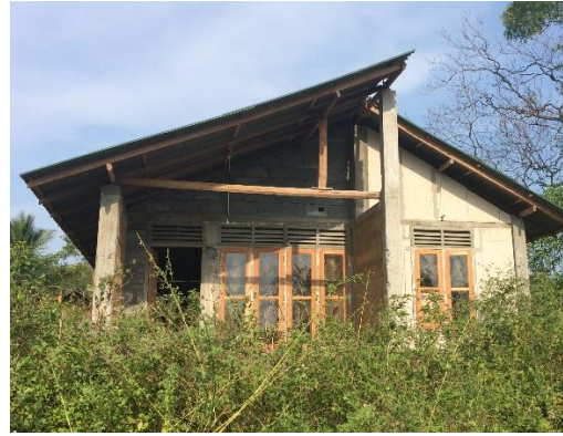
Figure 4-10: Model house: without plastering.
