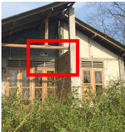
Figure 4-14: Rear side of real scale model house Actual Image, the red coloured area was captured by thermal camera.
