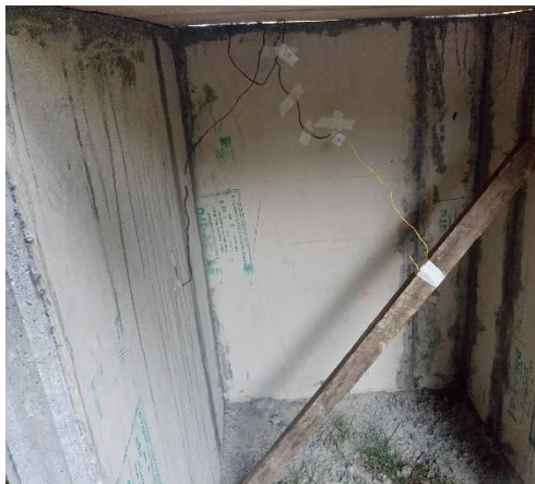
Figure 3-13: Installing the data loggers & connections
