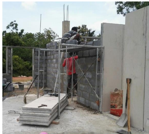
Figure 4-8: Construction phase: the model house has three different materials
