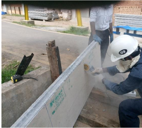
Figure 3-9: Reshaping the wall panels.
