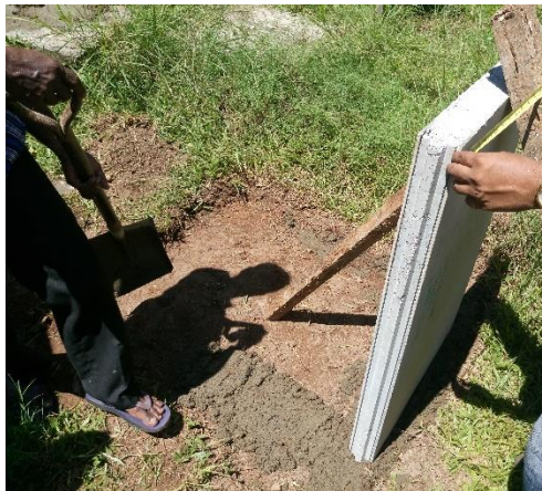
Figure 3-11: Initialize the wall panels
