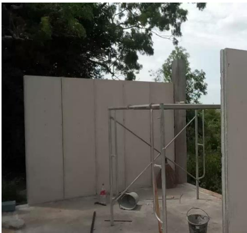
Figure 4-7: Construction Phase at Yayawatta, Tangalle
