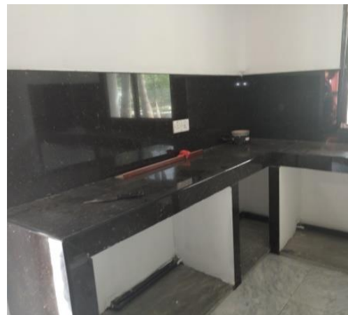
Figure 4-24: Kitchen Area (East Side)
