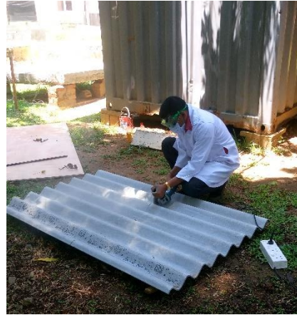
Figure 3-10: Reshaping the roof
