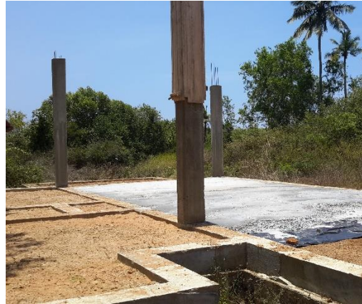
Figure 4-4: Completion of the foundation
