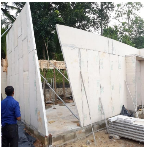
Figure 4-5: Similar house constructed by using wall panels.
