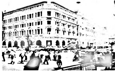
Figure 24-historical built fabric of York Street.
