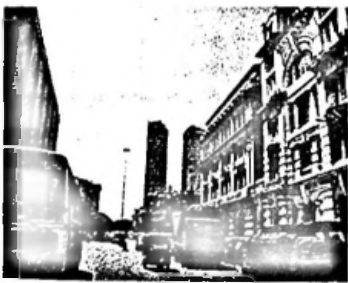
(Fig 155) View towards the high risers from the Port Authority Building
