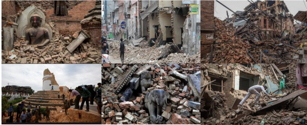
Figure 1.1: Damaged structures due to Nepal earthquake in 2015
