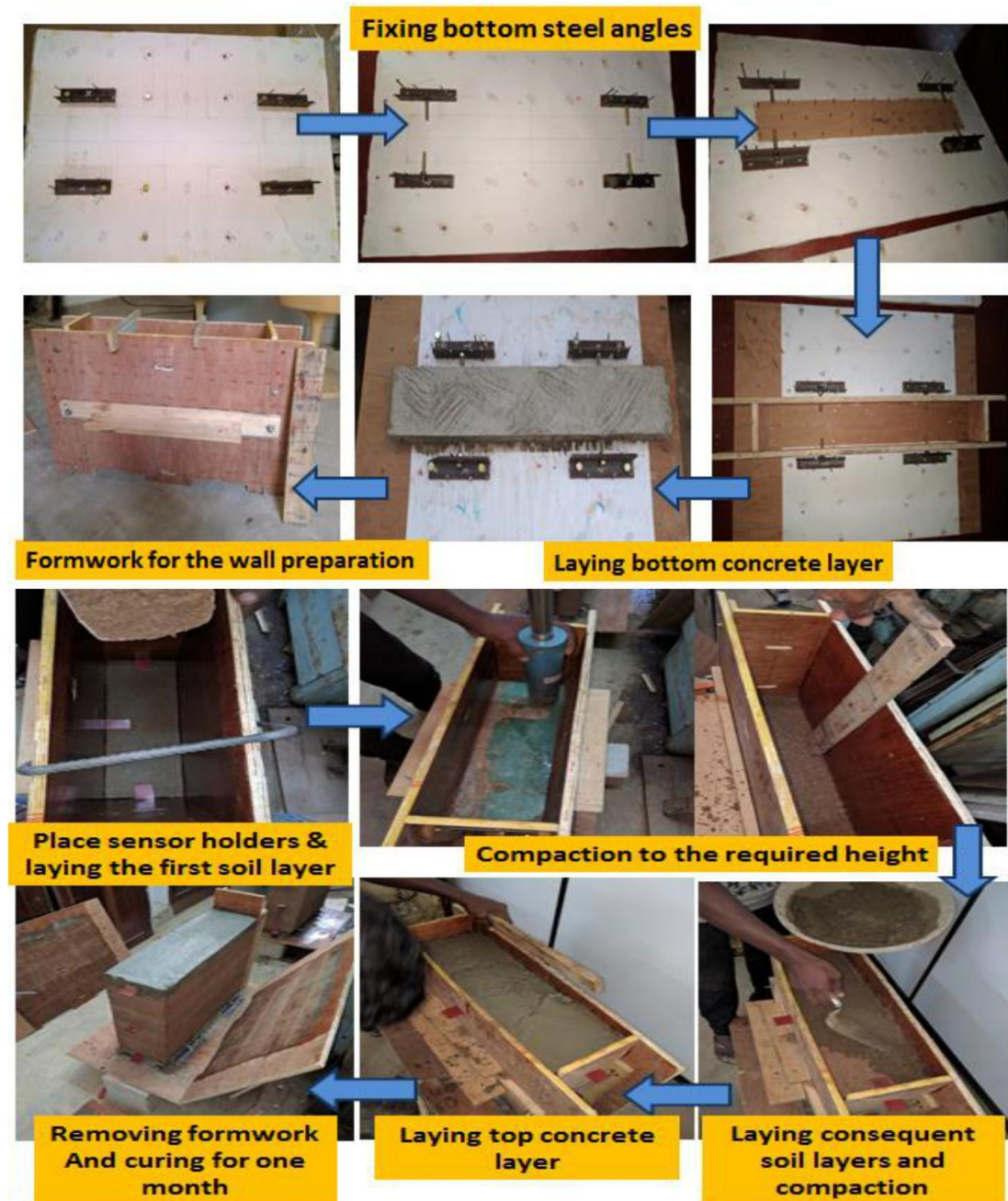
Figure 3.8: Construction steps of CSRE wall panels
