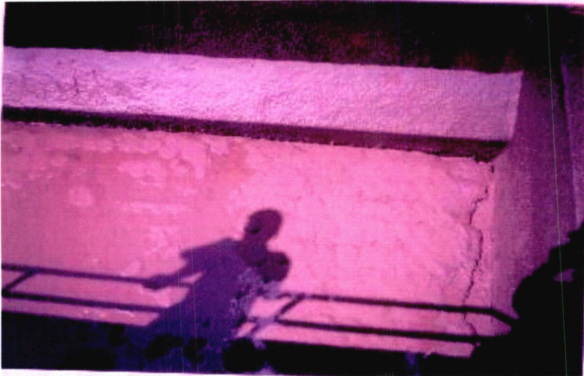
Fig. 2.15 Collection of floc on the filter bed
