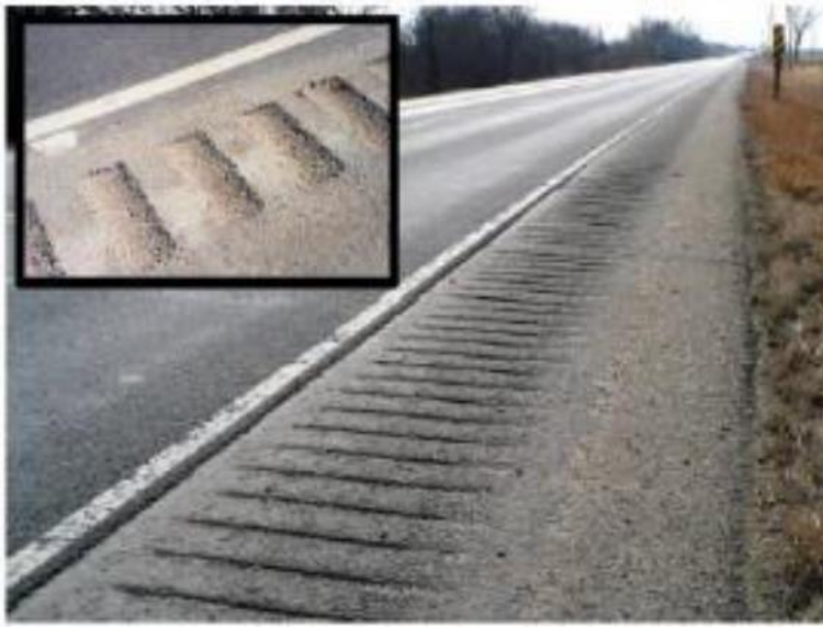
Figure 6.3: Rumble strips along the shoulder
