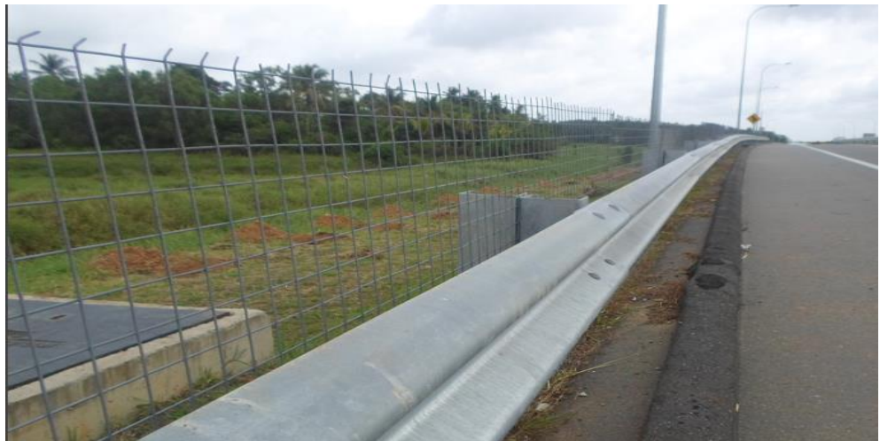
Figure 6.2: Secondary fence along with embankment guardrail
