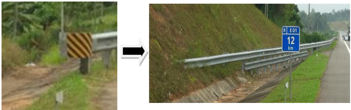
Figure 6.4: Re-arrangement of embankment guardrails
