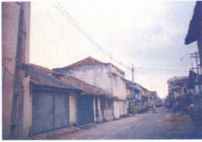
Fig. 34 The monotony of the Peddler Street. Lost the quality of residential scaled street. Disharmony can be experienced.
