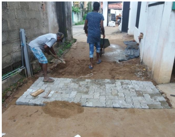
Figure 22- Constructing other sections (Block layer)
