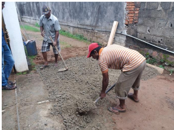
Figure 18- Ground preparation for Asphalt and primed sections
