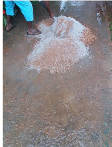
Figure 21- Dry mixing cement and soil for Mud Concrete
