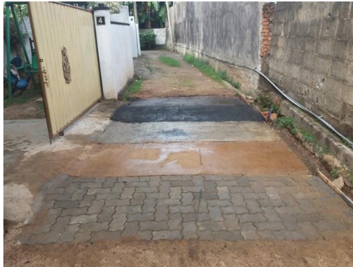
Figure 16- Prepared road section
