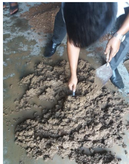
Figure 12- Cement and soil mixing
