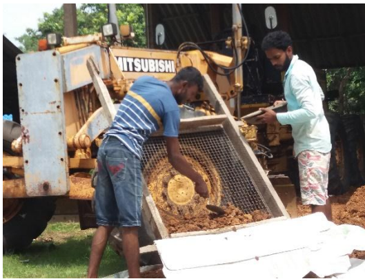
Figure 11- Removing boulder and debris by sieving through 20mm sieve
