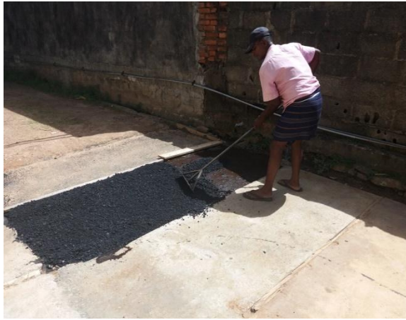
Figure 20- Constructing other sections (Asphalt layer)
