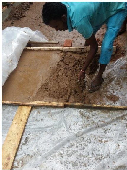
Figure 23-Preparing of Mud Concrete layer
