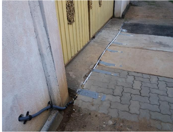
Figure 24-Installation of thermal sensors
