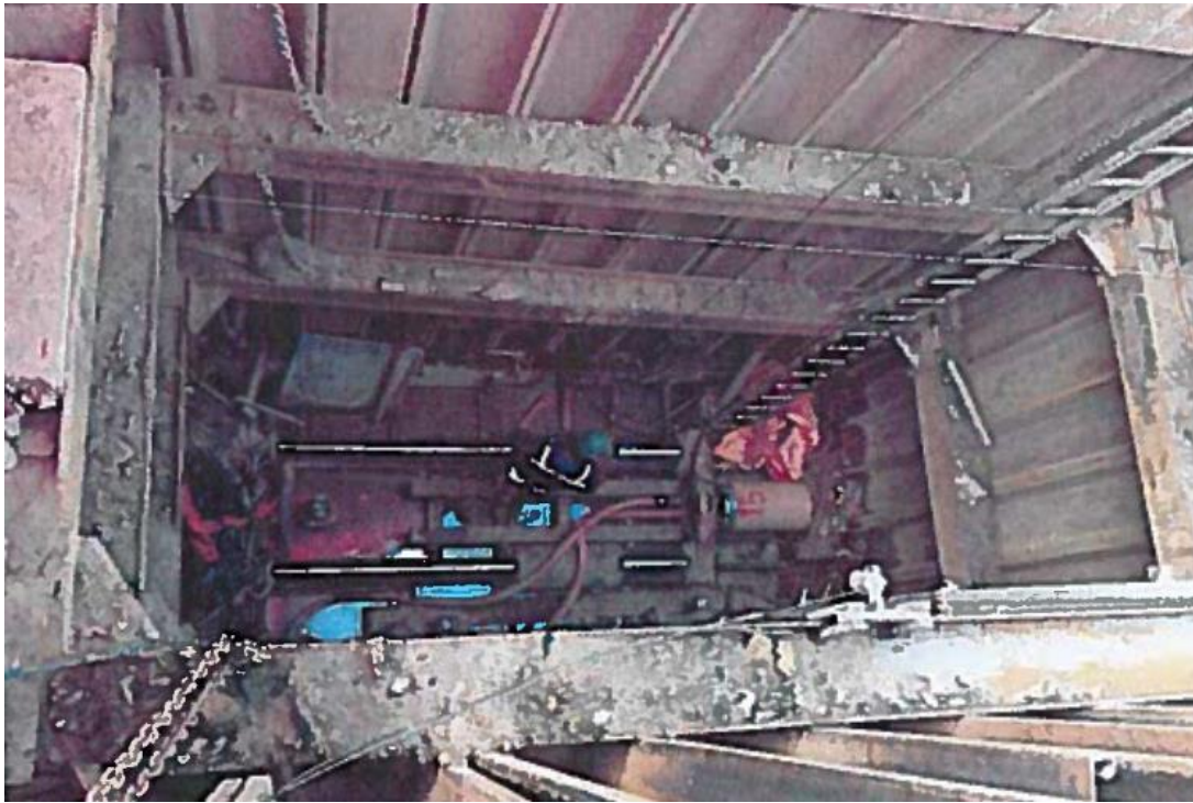
Figure 40 - VC pipe Jacking in operation
