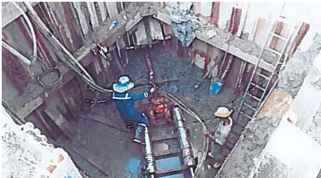
Figure 41 - Jacking of steering head and pilot tubes from jacking pit
