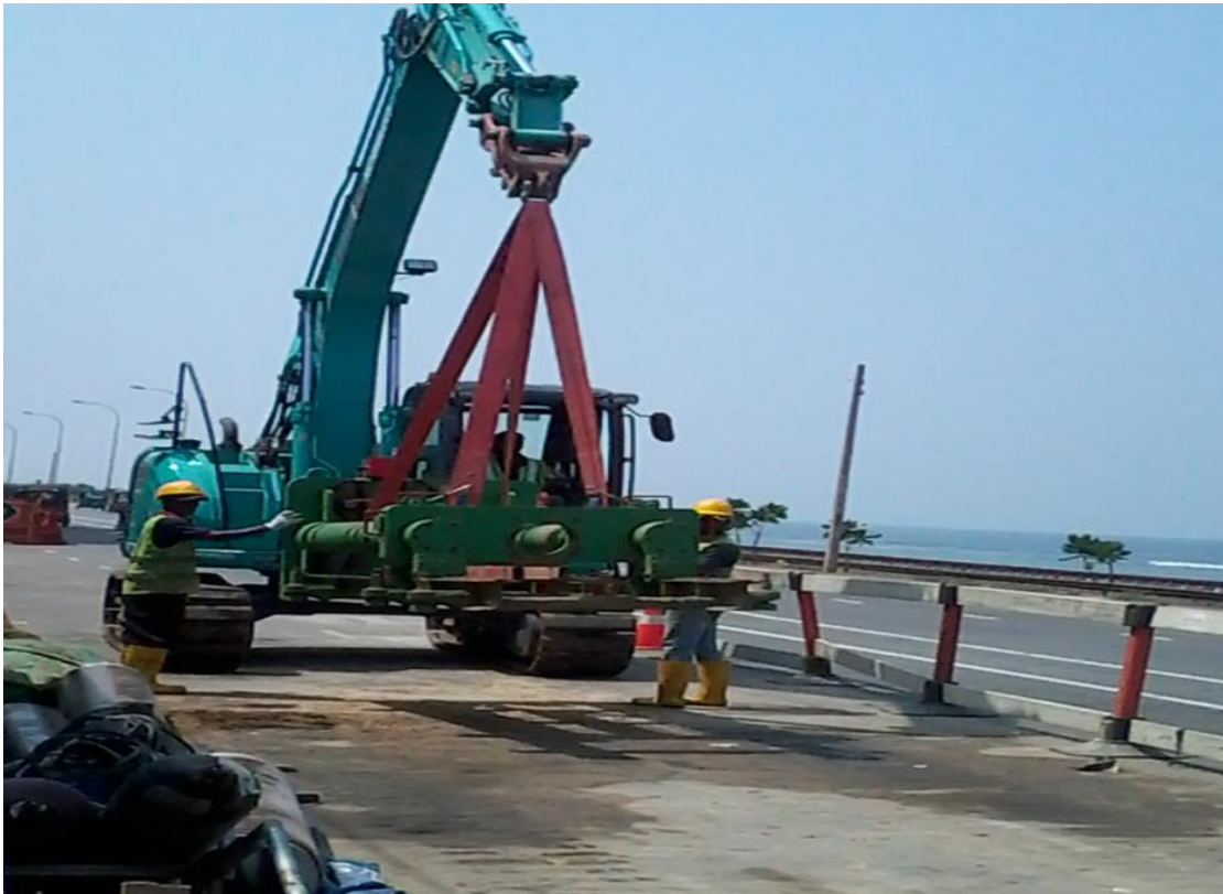
Figure 31 -Carryover of TBM from one place to another
