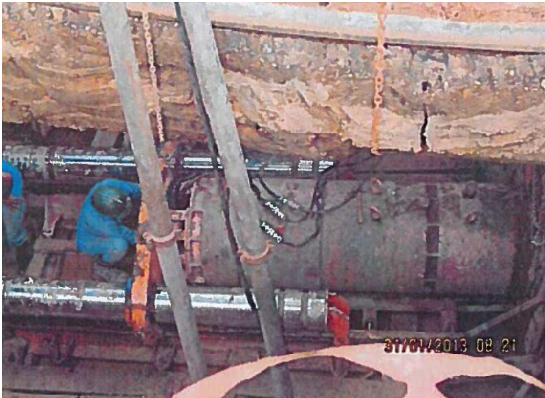
Figure 38 - Jacking of TBM Shield
