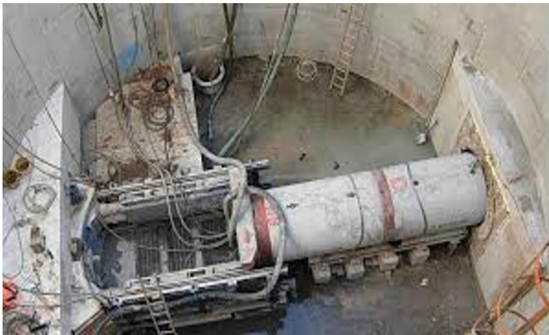
Figure 16 -Typical arrangement of microtunneling jacking shaft
