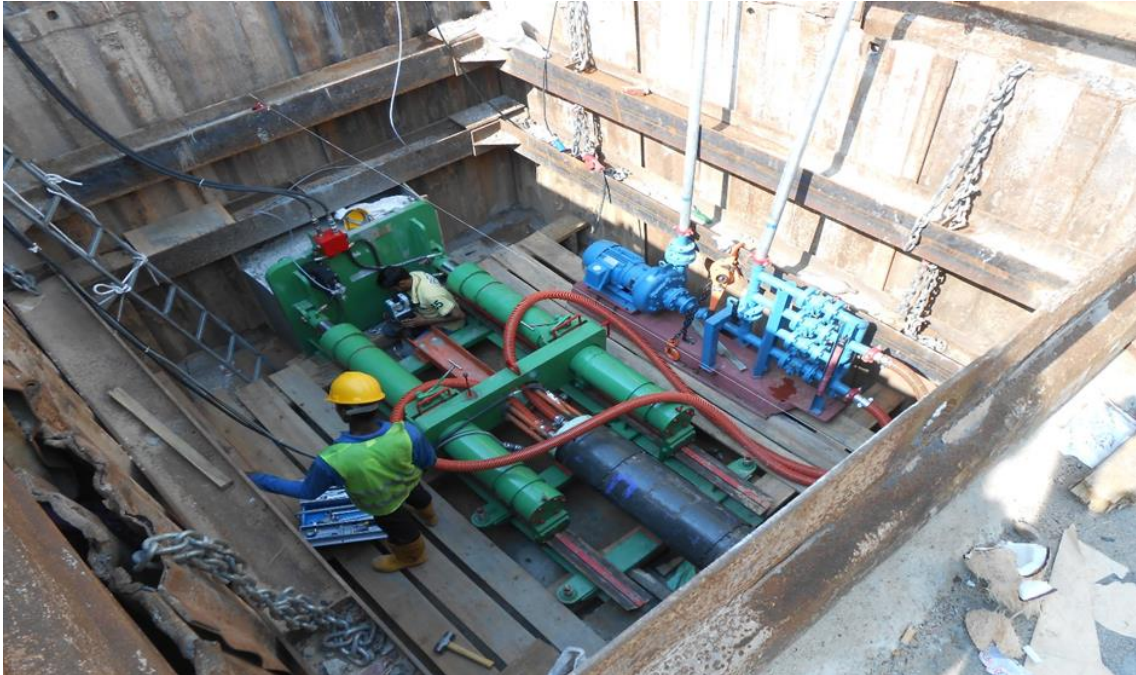
Figure 33 - Checking the pipe alignment
