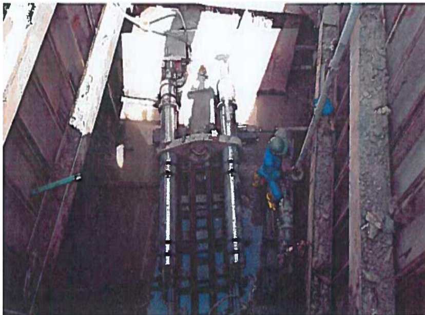
Figure 36 - setting-up of guide rails and jacking rig
