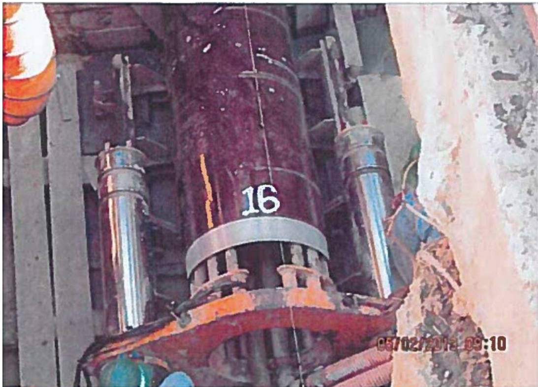
Figure 39 - Jacking of product pipe
