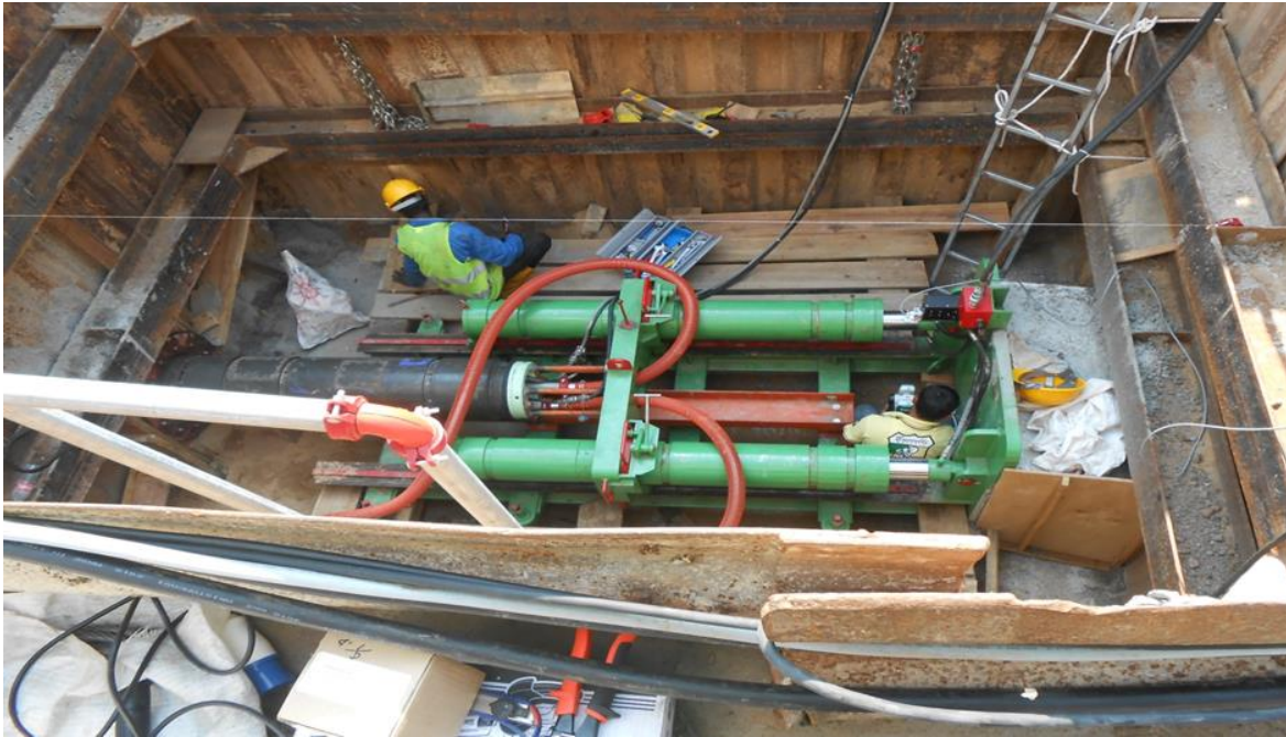
Figure 30 Jacking machine is in operation
