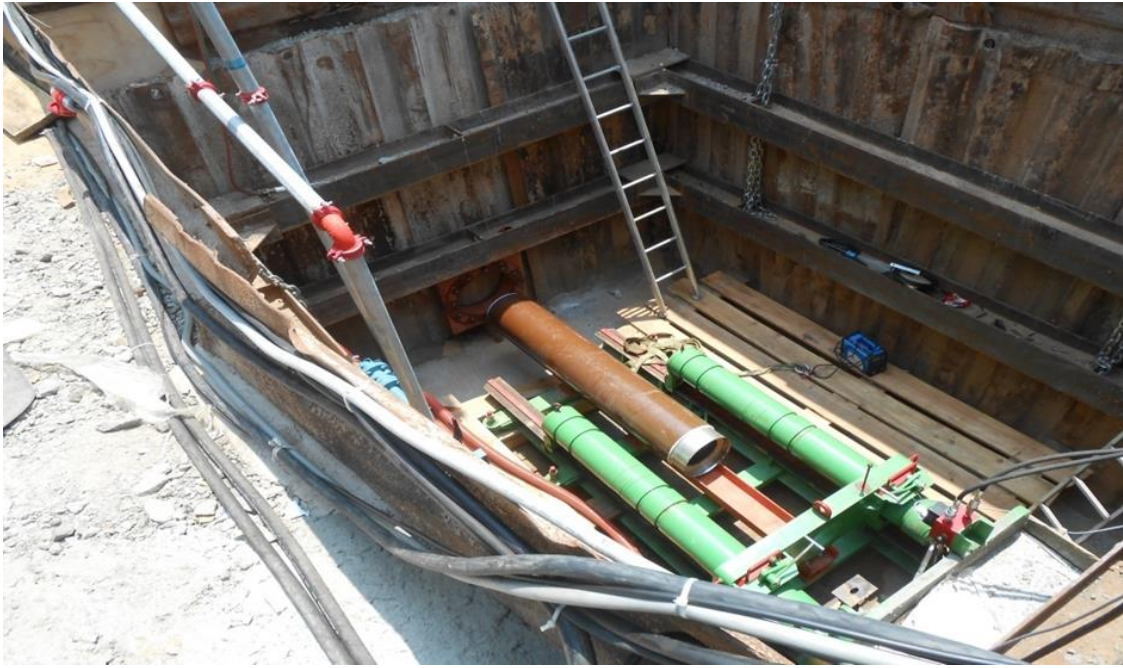
Figure 32 - Preparation of driving shaft at Manhole No.18
