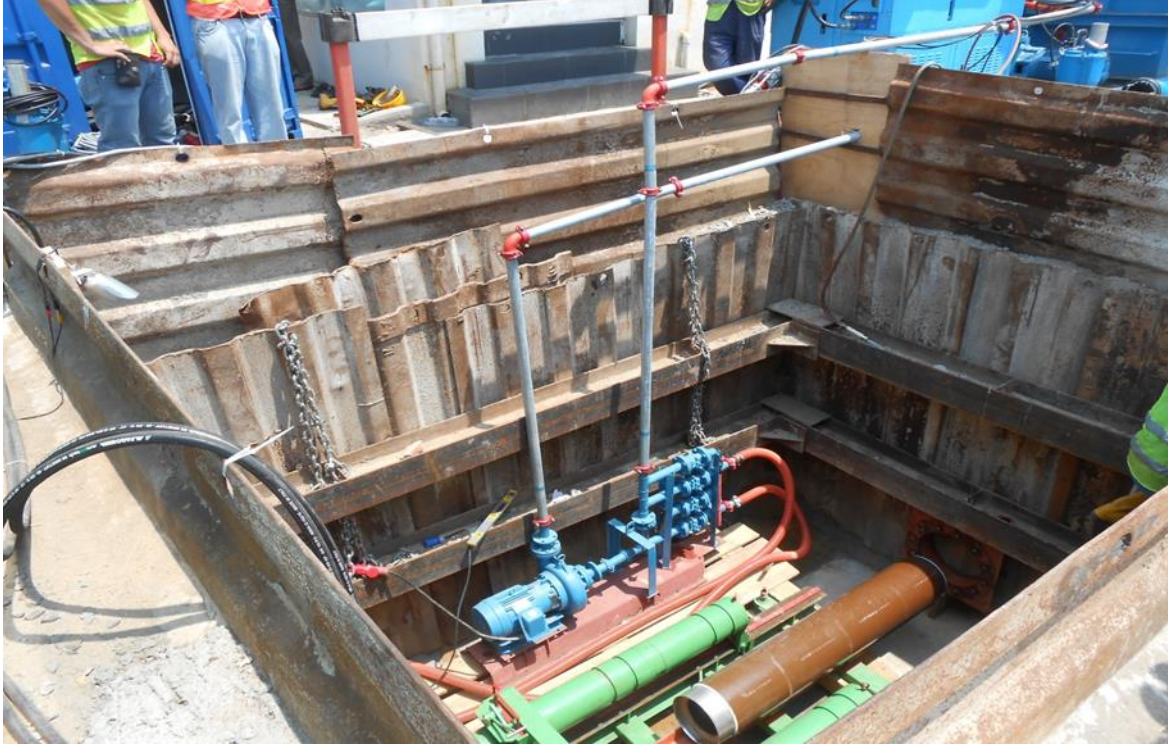
Figure 29 Installation of Jacking Machine
