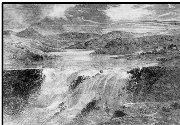
Figure 1-1- Dale Dike Dam failure (Brownjohn, 2007)
