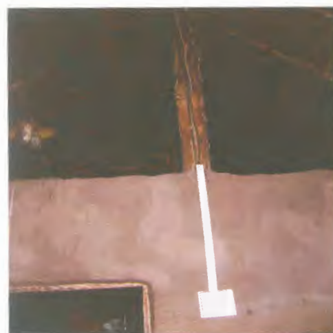
Wiring on Walls & Roof Rafters
