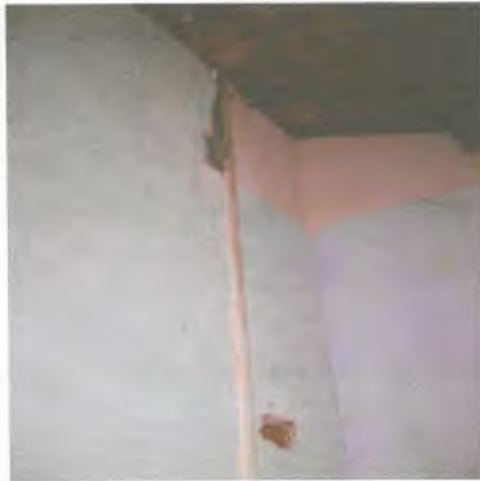
Wiring on Walls & Roof Rafters
