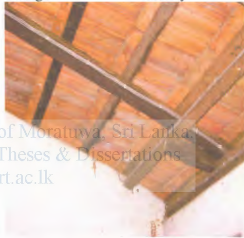
Wiring on Roof Rafters
