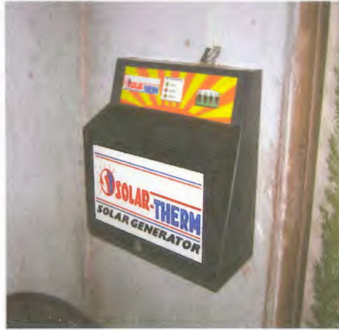
Charge Controller & Battery Box
