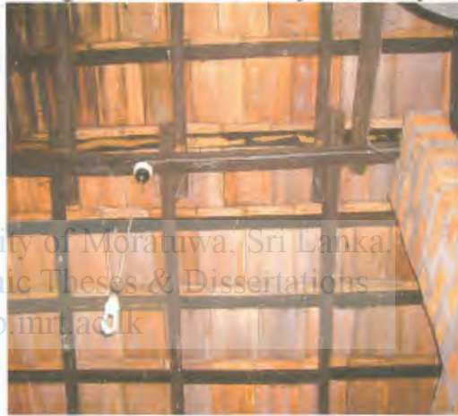
Wiring on Roof Rafters
