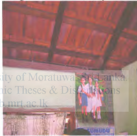
Wiring on Roof Rafters
