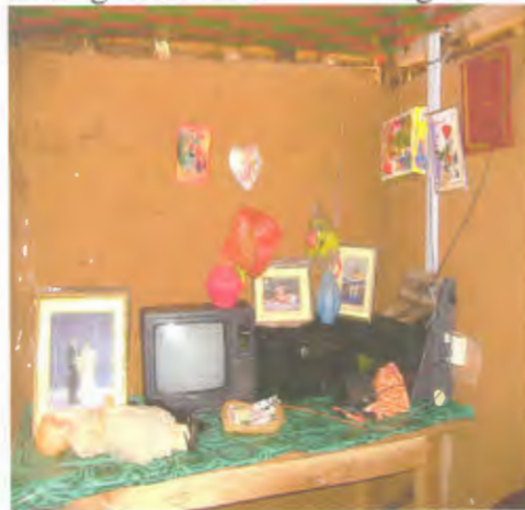
Wiring on Walls Surface
