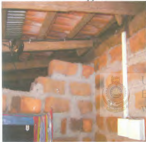
Wiring on Roof Rafters
