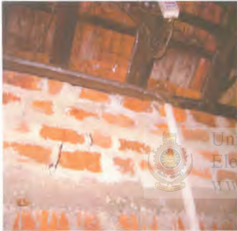
Wiring on Walls & Roof Rafters
