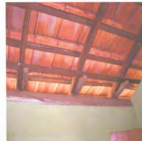
Wiring on Roof Rafters
