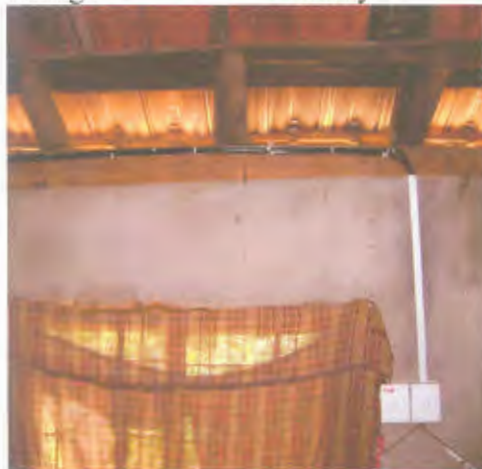
Wiring on Roof Rafters
