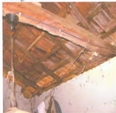
Wiring on Roof Rafters
