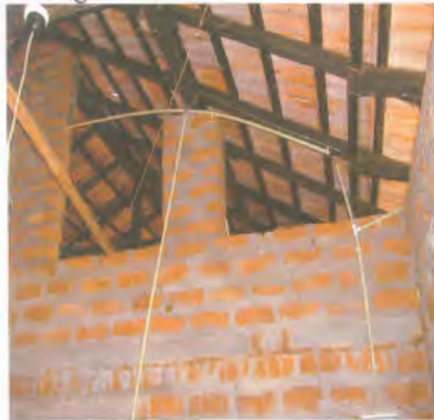
Wiring on Walls & Roof Rafters
