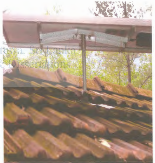
Figure 3.3.1: Pictures Depicting Module Support Structures
