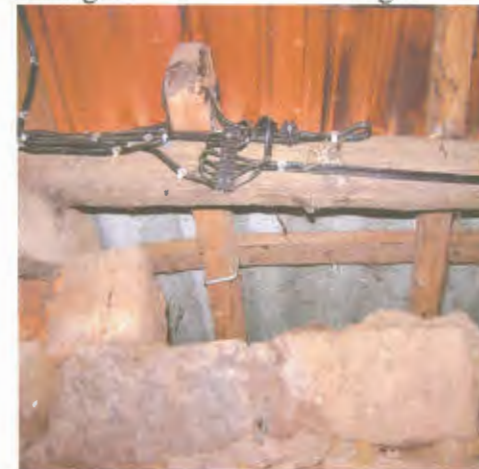
Wiring on Roof Rafters
