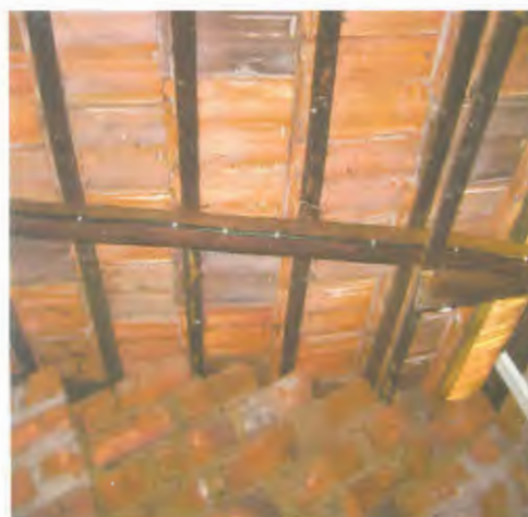
Wiring on Roof Rafters
