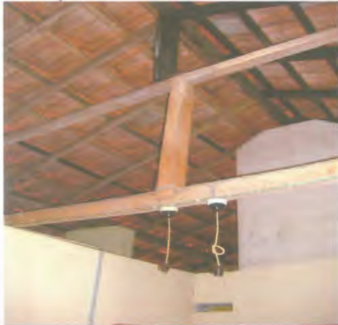
Wiring on Roof Rafters
