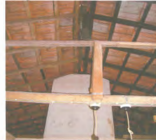
Wiring on Roof Rafters
