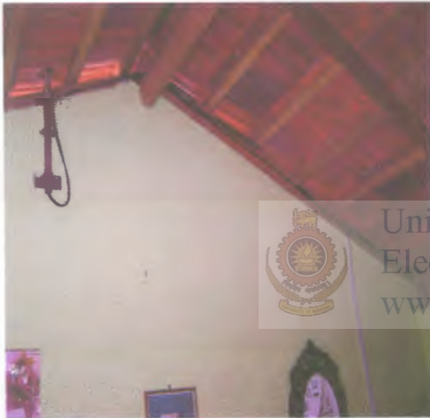
Wiring on Roof Rafters
