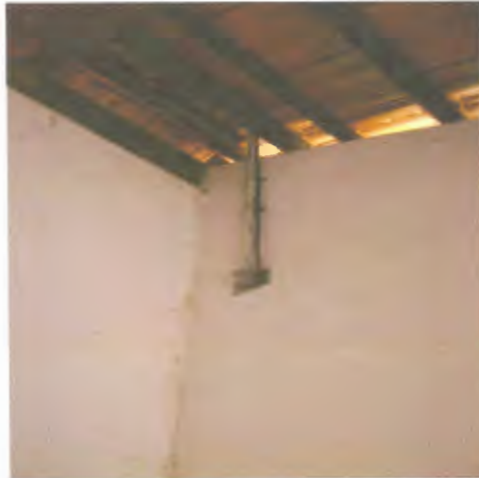
Wiring on Roof Rafters
