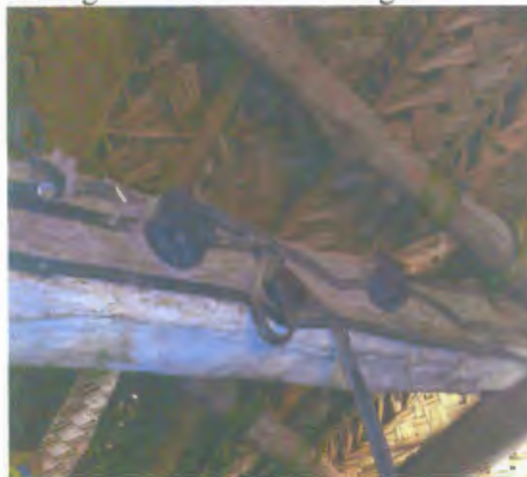
Wiring on Roof Rafters
