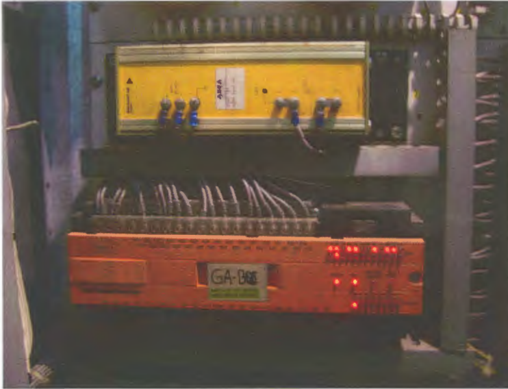
Figure 3.4.1 Basic unit of the BSC controller (MasterPiece 020)
