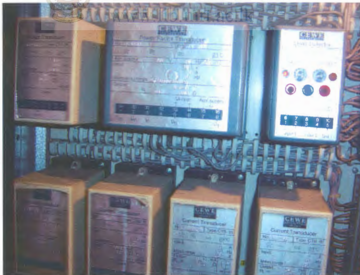
Figure 3.4.2 Type of the transducers used for the signalling
