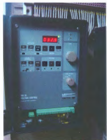
Figure 2.5.2 Front view of the modern MR Tapcon 260 AVR control relay and MK 30 relay
