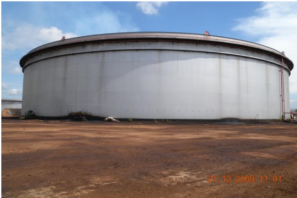
Figure 4. 1 Practical size of a Refinery Floating roof Crude oil tank in Refinery
