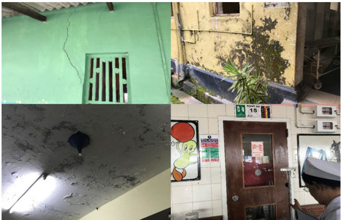
▼ Figure 3: Pictures captured during the rapid visual inspections in hospitals
