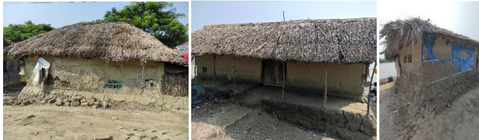
Figure 3, Elevation of mud house (left), semi-private “dawakhana” (verandah) outside main house (middle), high plinth to withstand flood (right) (Source- Author)
