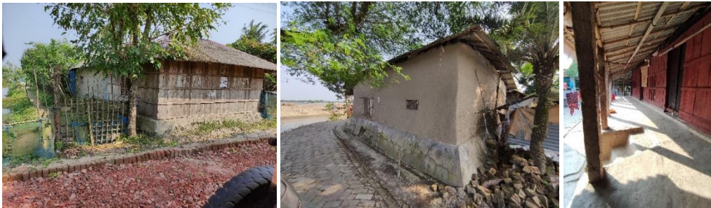
Figure 4, Mud plinth covered with cement and wooden walls (left), mud plinth covered with cement and mud walls (middle), mud plinth and wooden walls (right) (Source- Author)
