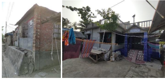
Figure 5, Brick building with columns (Source- Author)
