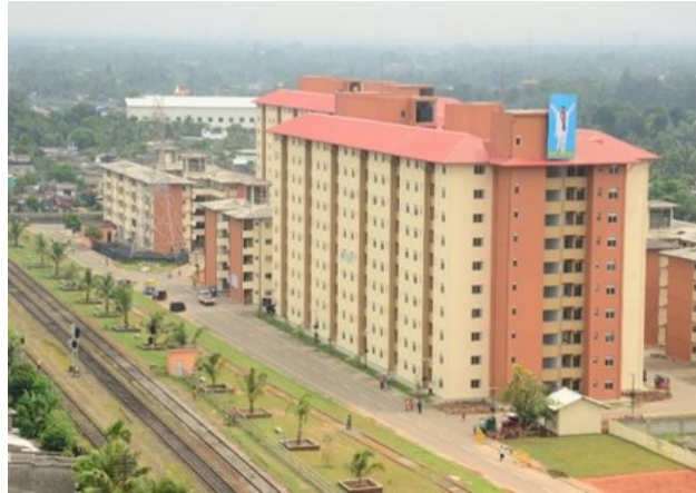
Figure 4-1: Birds eye view of the relocation houses
