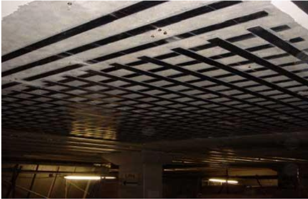
Figure 4: Slab strengthening using CFRP laminates (Chowdru & Islam, 2014)
