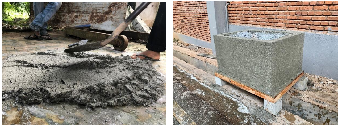
Figure 81. Application of EPS plaster as external wall plaster
