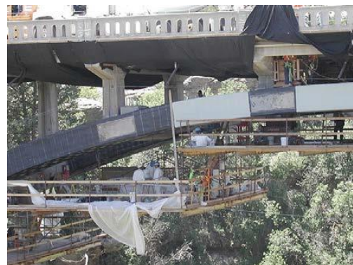
Figure 7: Concrete bridge retrofitted using CFRP sheets (Sonnenschein, Gajdosova, & Holly, 2016)
