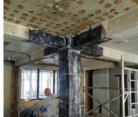
Figure 5: Strengthening of Beam-Column joint using CFRP (Chowdru & Islam, 2014)
