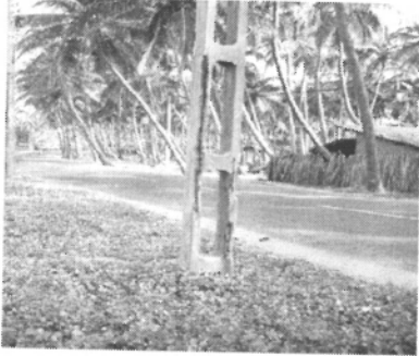
Fig.5.5: Corroded concrete poles at coastal areas
