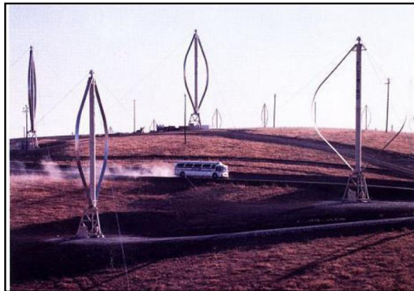
Figure 13: Wind Farm under FloWind
