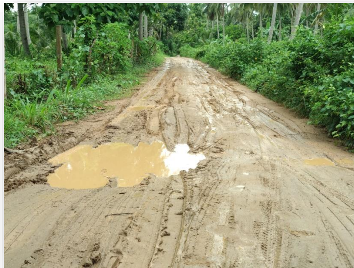
Figure 1.2:Gravel road in the rainy season
