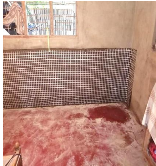
(d) Application of scratch coat and epoxied geogrid
