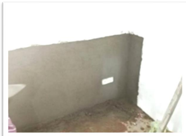
(e) Final coat of rendering after embedding the geogrid
