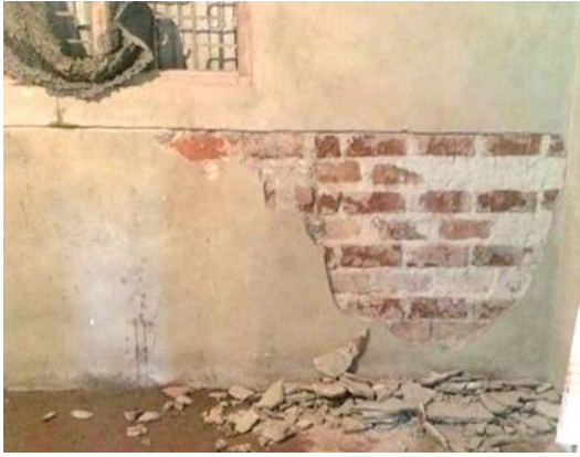
(a) Removal of existing plaster
