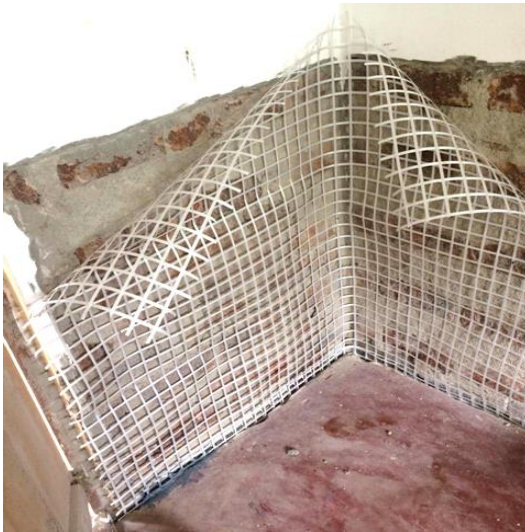
(c) Curing of epoxy
