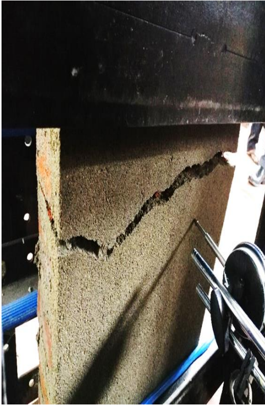
Horizontal flexural crack
