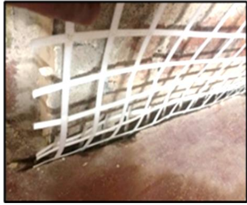
(b) Epoxy the geogrid in place
