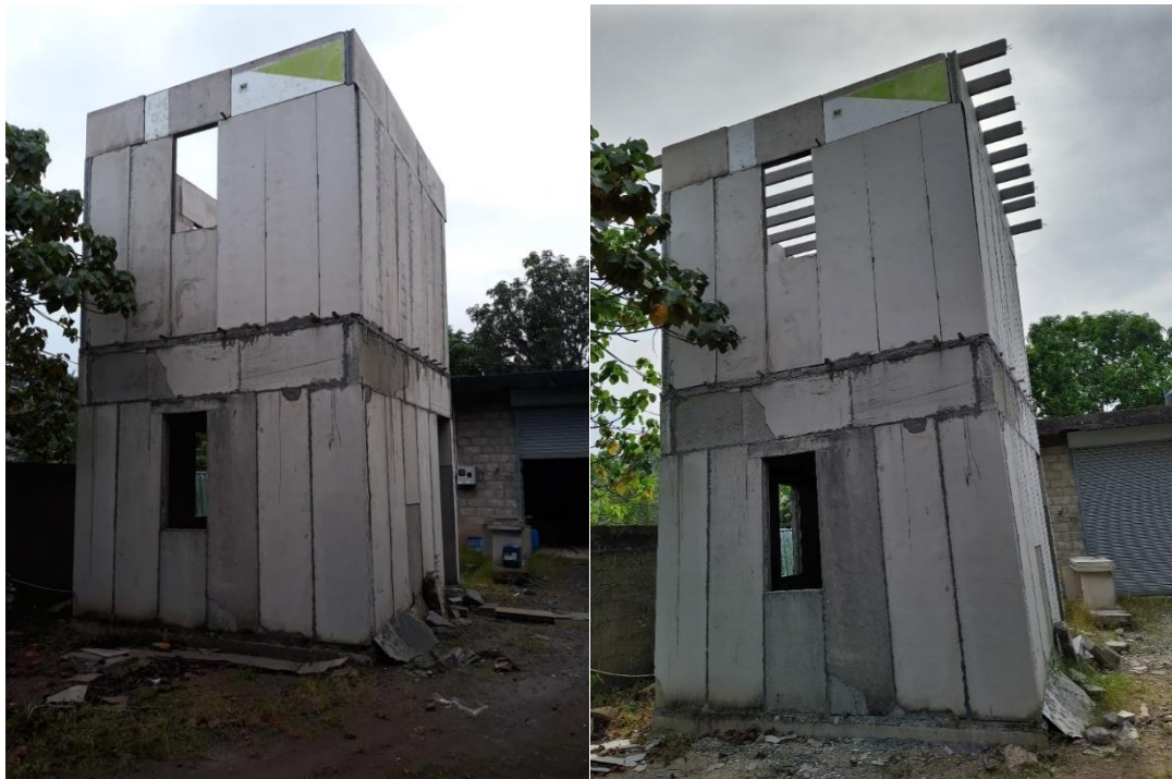
Figure 37: LWC panel based Refuge space construction
