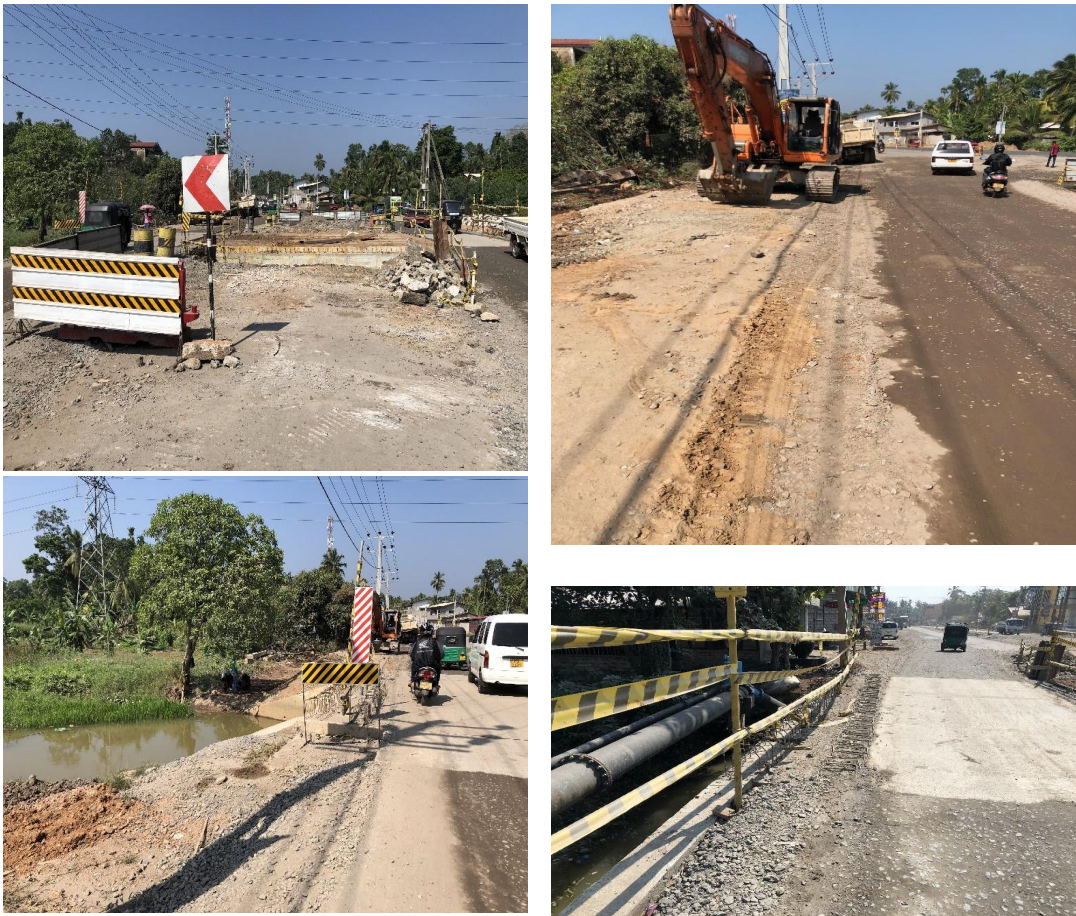
Figure 9: Culvert construction site
