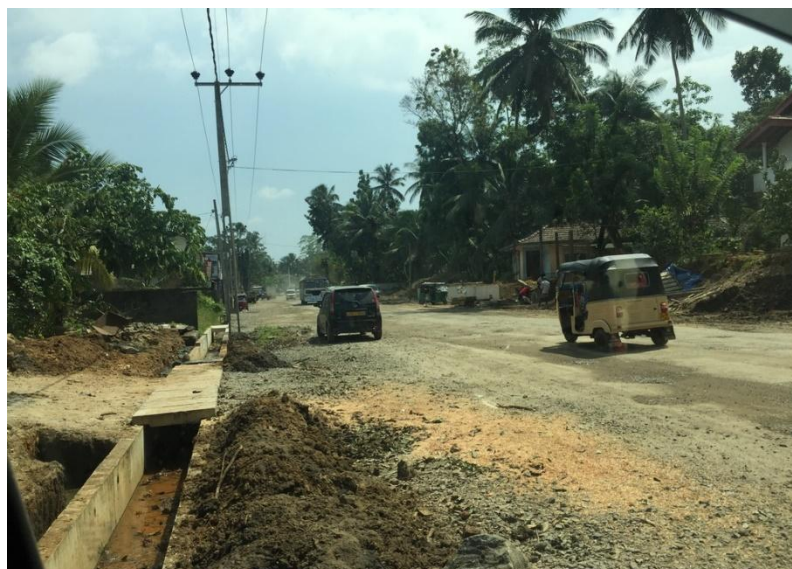
Figure 2 Temporary road way in road construction zone in Sri Lanka
