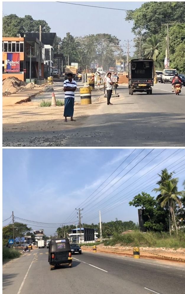
Figure 15: Pavement construction and widening
