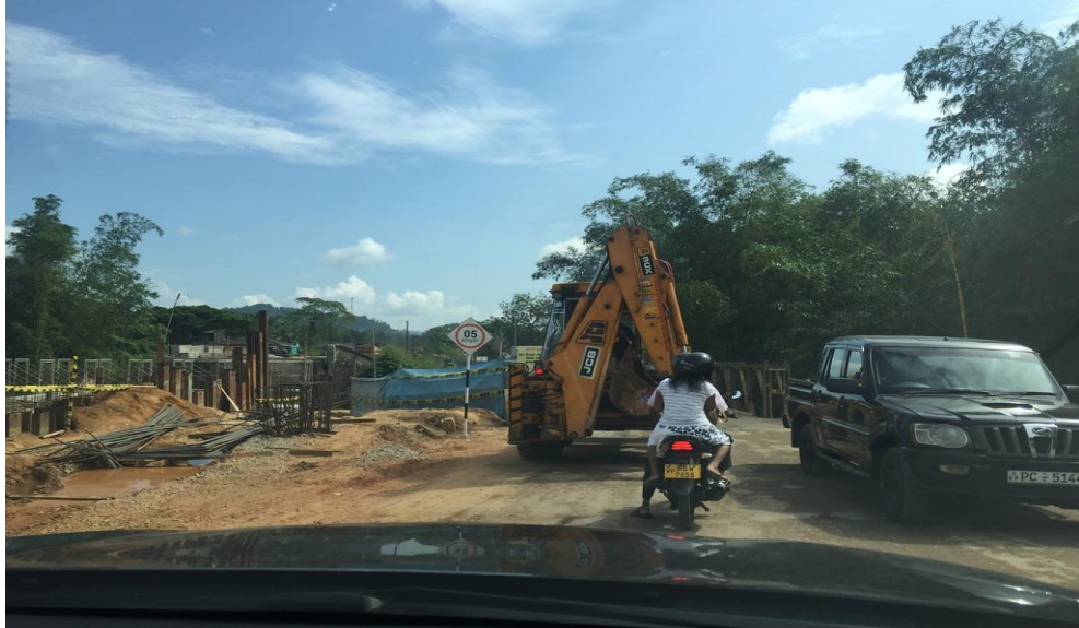
Figure 19: Bridge work zone
