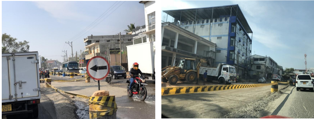
Figure 17: Work zone near Yakkala Junction
