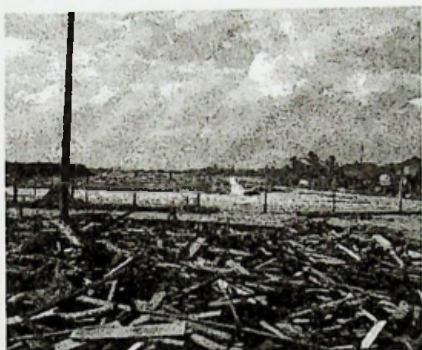
Fig.4: Severe infrastructure damage to the salton
