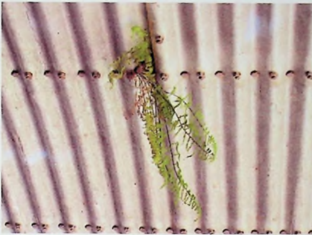
Figure 3.2 : Weeds comes through the plates of Metal Structure.
