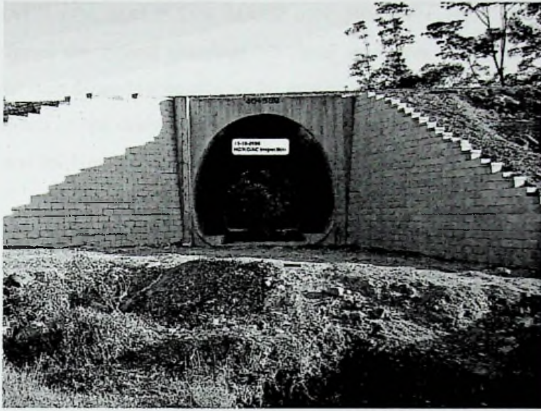
Figure 1.1 : View of a Metal Structure
