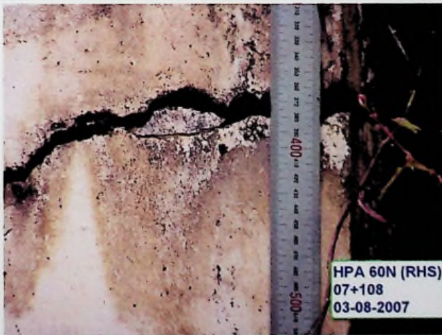
Figure 3.1 : Husker walls are cracked.
