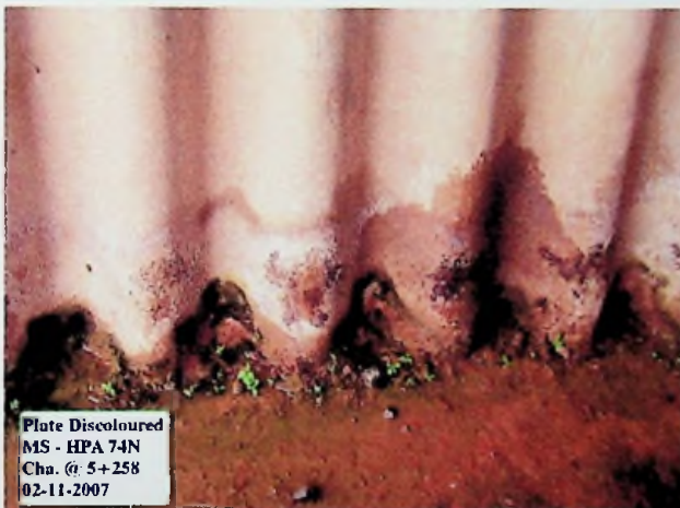
Figure 3.3 : Plates are Corroded..
