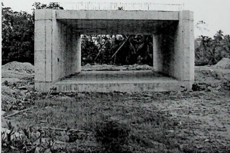
Figure 1.2 : View of a Box Culvert
