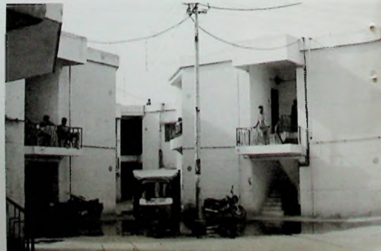
Image 28: Blank walls define the public space of the street, which serves primarily as a conduit for vehicular circulation. Private balconies afford little opportunity for interaction with neighbours.
