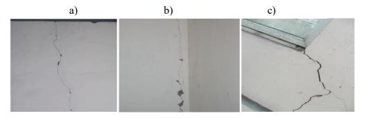
Figure 1: Types of cracks - a) thin crack, b) medium crack and c) wide crack Source: Kunal and Killemsetty (2014)
