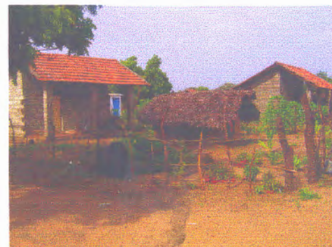
Fig. 113-Existing palm leave structure
