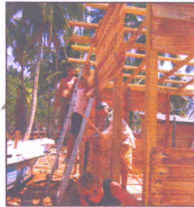
Fig. 58- Construction of wooden houses
