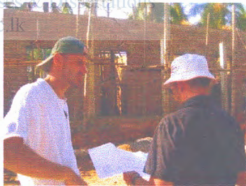
Fig.68- Medical centre at under construction
