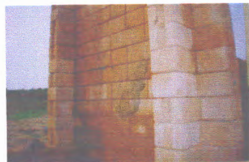
Fig. 42- Clay –cement brick wall
