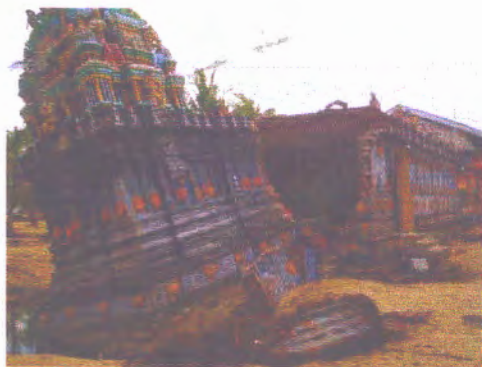
Fig. 80- Damaged Hindu Shrine
