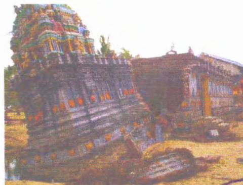
Fig. 16- Destroyed Hindu Temple in Ampara
