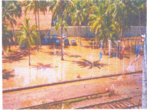
Fig.19- Flooded entrance of Blue water hotel
