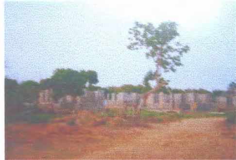
Fig. 100- houses are in same under construction stage
