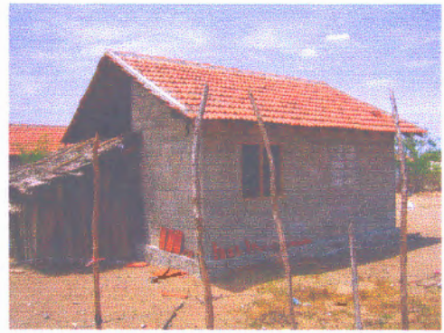
Fig.114 - Addition of outside kitchen
