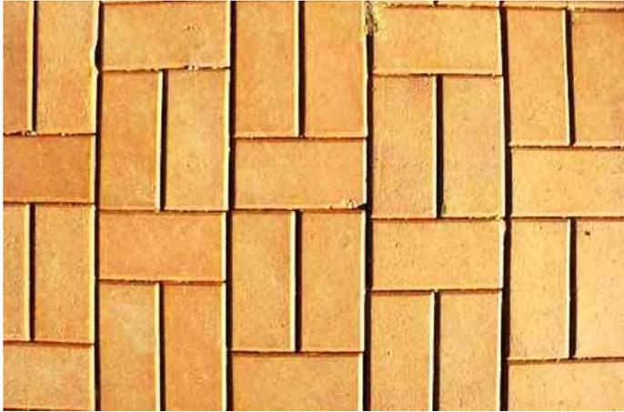
Figure 15: Mud concrete paved area.
