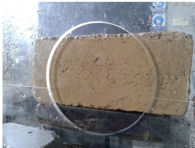
Fig. 17. No significant cavities were visible in tested sample of MCB after carrying out the accelerated erosion test.
