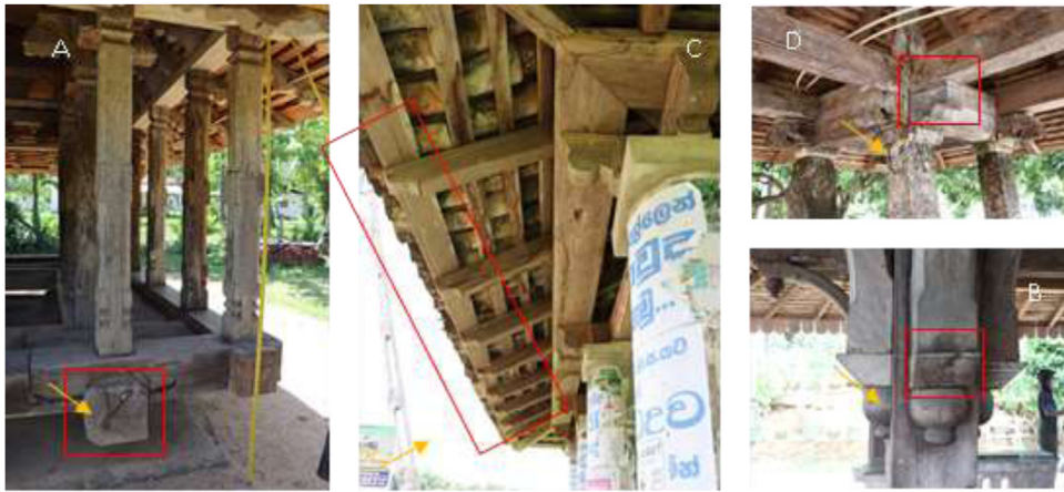
Fig. 7. A: Panavitiya Ambalama (bearer); B: Badulla Ambalama; C and D – Giruwa Ambalama (king rafter, rafter, bearers).
