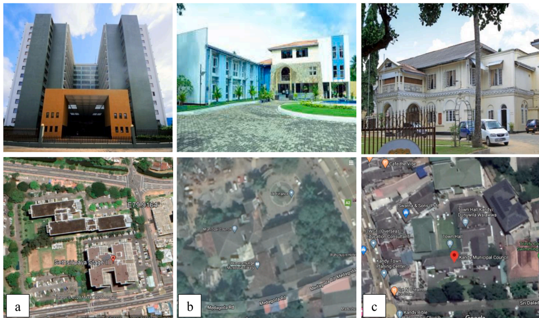
Fig. 2. Selected buildings a) Colombo Sethsiripaya b) Matara urban council c) Kandy urban council.
