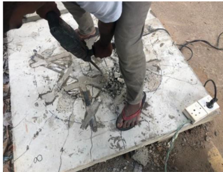
Fig. 4. Drilling the damaged concrete area.
